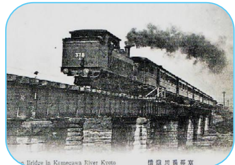
Bridge in Kamogawa River Kyoto
